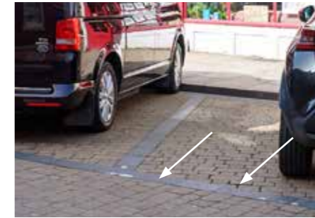
Parking Bays - Black basalt setts
