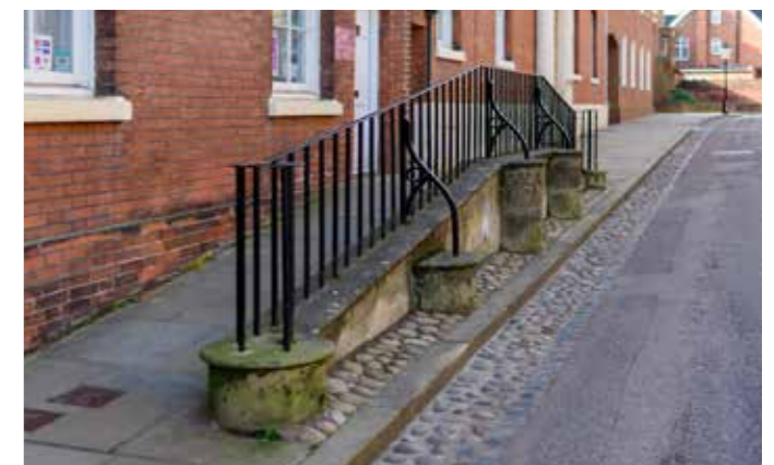
Railing detail: Cathedral Close (above)
