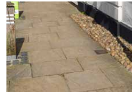
Footpath - Yorkstone to west of junction
