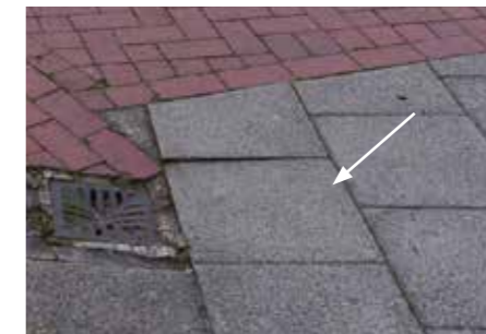
Footpaths - PCC flags to south west
