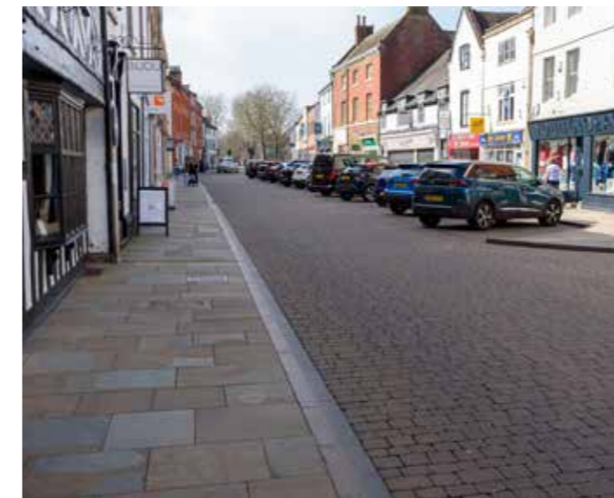
Natural stone paving and tegula carriageway on Bore Street
