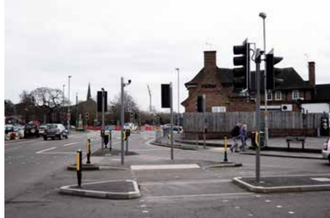
Vehicle and road infrastructure dominate Greenhill
