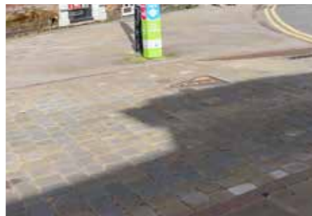
Highway - Transitions yorkstone setts
