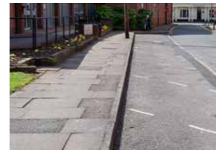
Footpaths - 400 x 400 concrete slabs (north)
