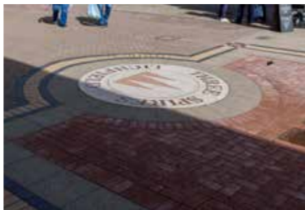
Footpath - PCC flags within arcade
