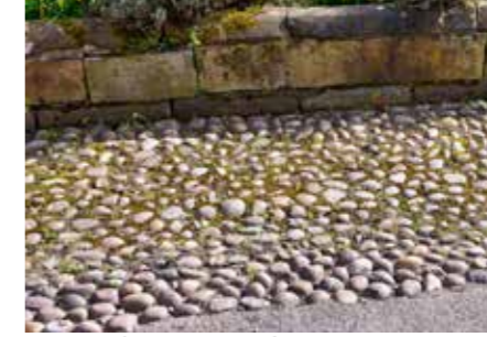
Back of paving/infill - Cobble on edge detail
