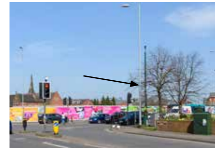
Lighting - 10m highway lighting columns
