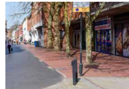
Footpaths - Red brick (stretcher) to arcade
