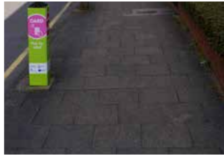
Footpaths - 400 x 400 concrete slabs
