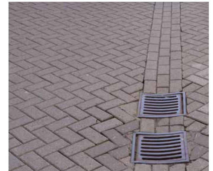
Concrete block paving on Bore Street (east)
