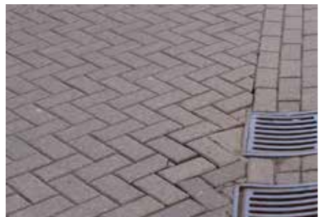
Highway - Concrete paviours (herringbone)
