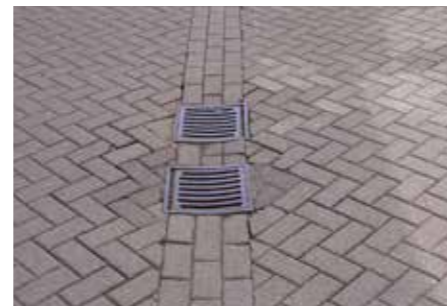
Channel - Concrete paviours (stretcher) central
