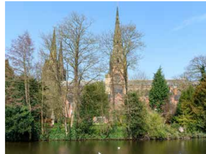
Filtered, not screened views of the cathedral (above)
