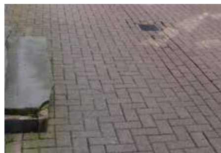
Highway - Buff concrete paviers (herringbone)
